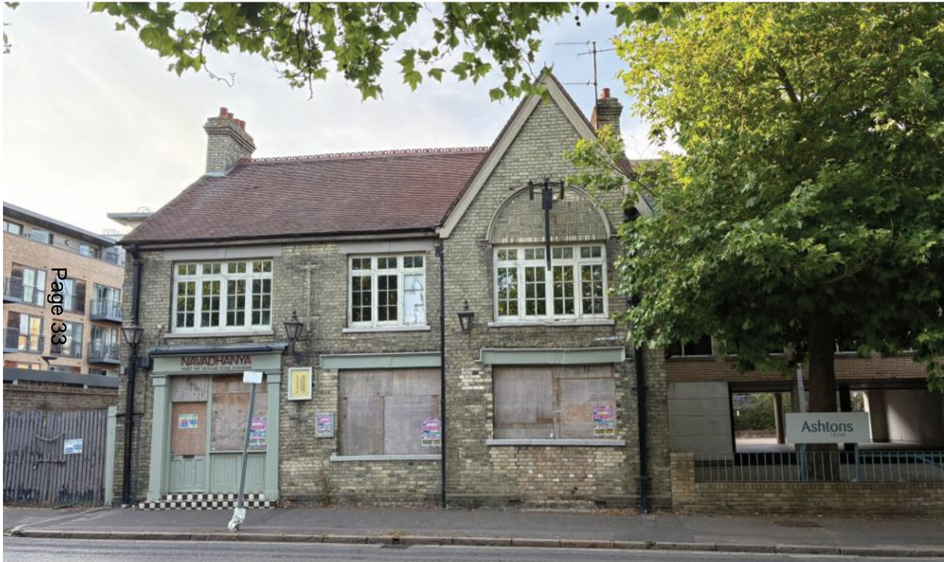
The existing building
